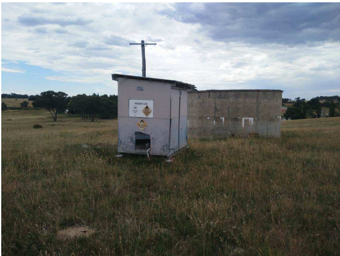
Plate 12: Pump-house with Likely Fibrous Cement Cladding – Sample TS10
