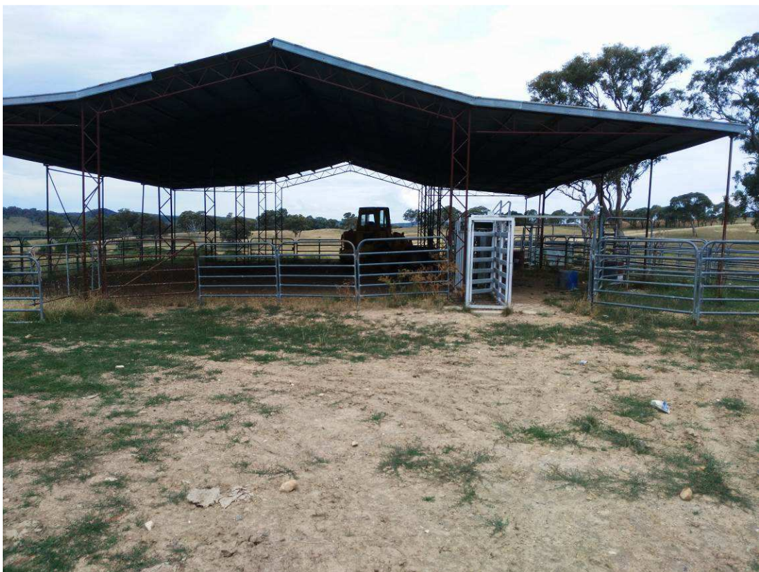
Plate 10: Machinery Shed – Sample TS6
