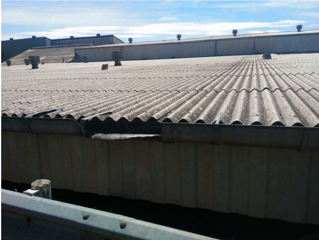
Plate 13: Roof of Abattoir Facility (Southern Portion) with Likely Fibrous Cement Sheetting
