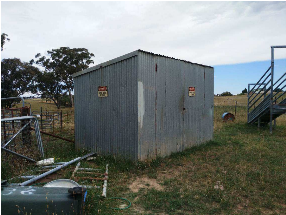
Plate 11: Flammable Goods Shed – Sample TS7
