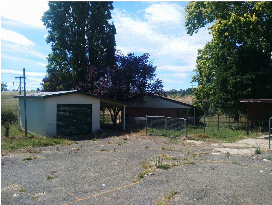
Plate 14: Structures Ancillary to Caretaker's Residence, with Likely Fibrous Cement Sheetting
